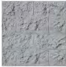
PAINTED SPLIT-FACE CMU
