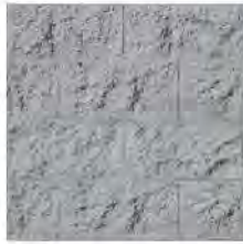
PAINTED SPLIT-FACE CMU
