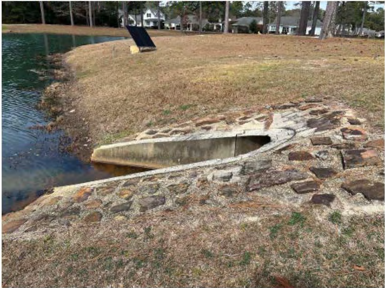
Outfall Pipe from Sweetwater Lake: No maintenance needed.
