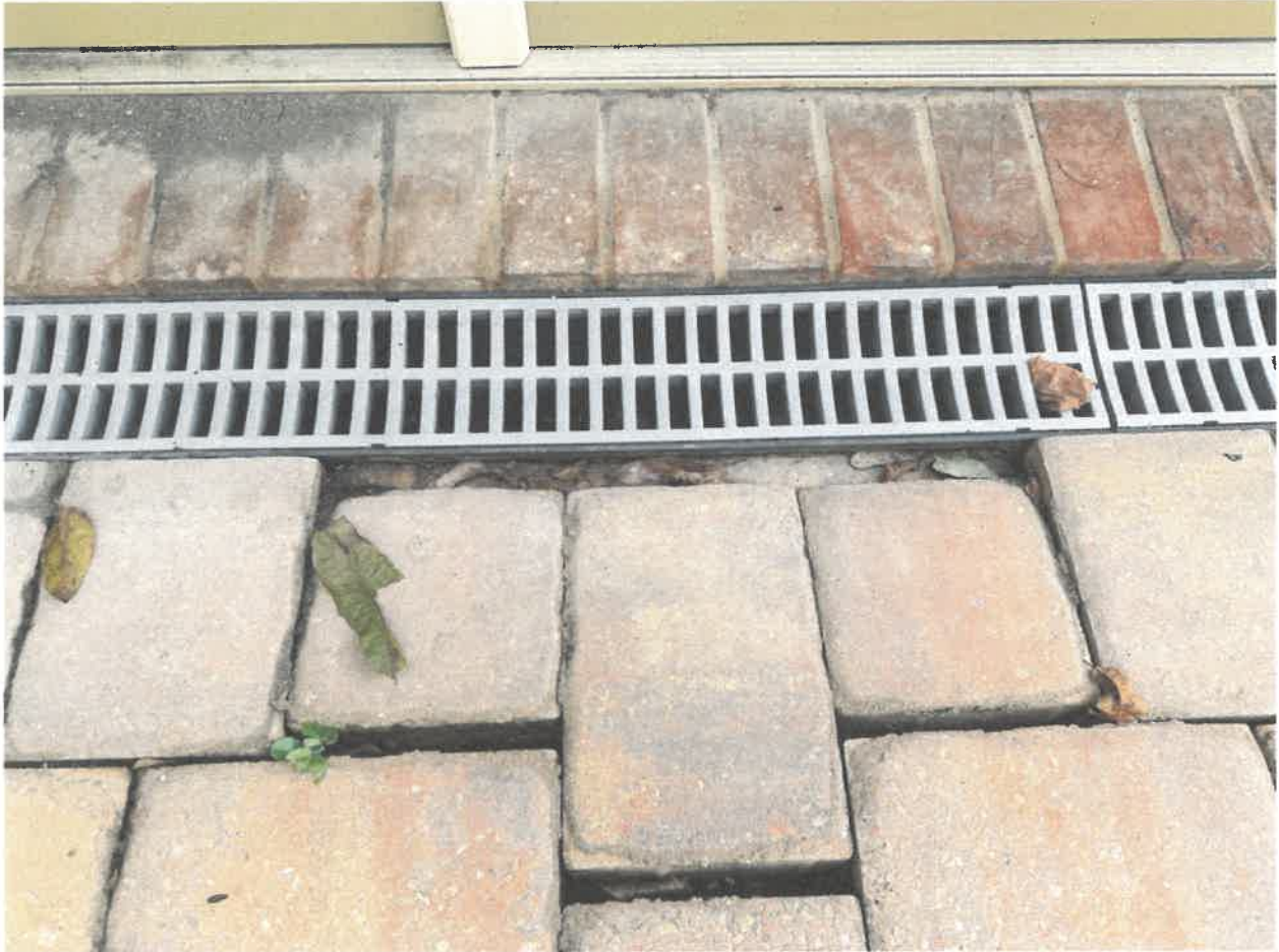
Erosion on west side of house.
