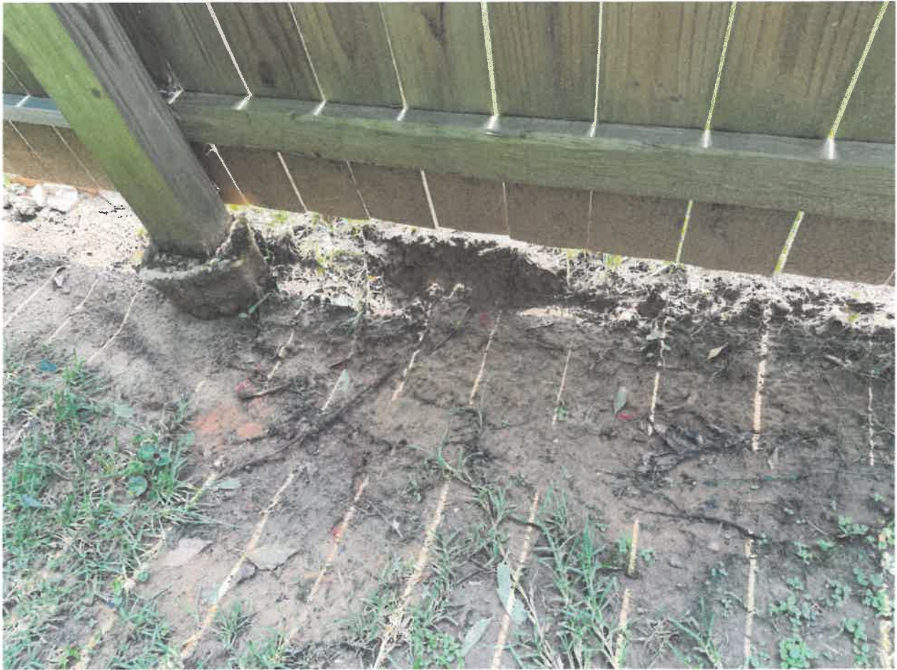
Erosion west of driveway pad.
