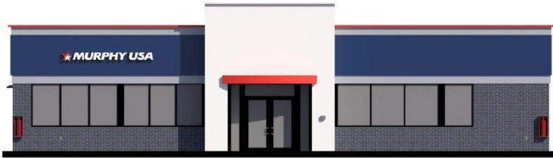
Figure 2: Front - Building Only (Facing South)
